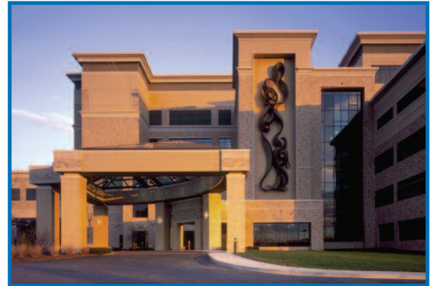
One of ETTI's recent projects was Central DuPage Hospital. It located utilities, conducted an infrared survey and performed a power quality analysis.
